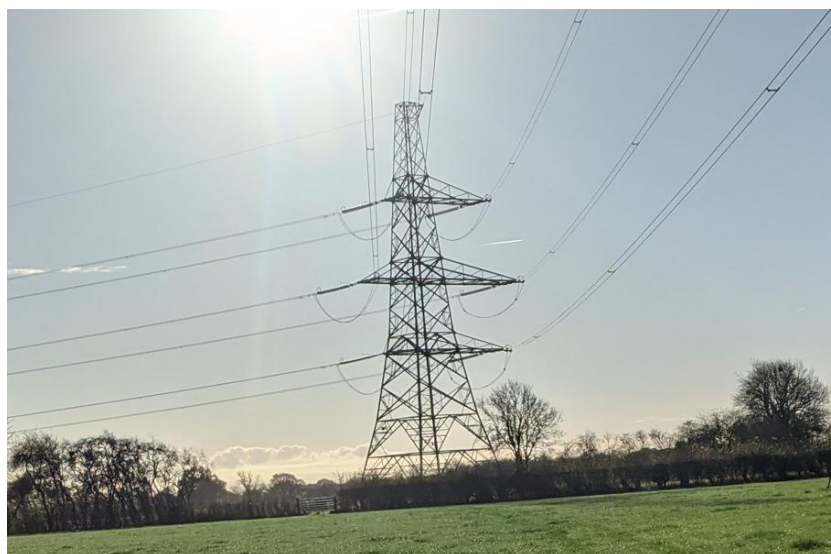
Image 5.12 Typical tension/angle lattice pylon 2
